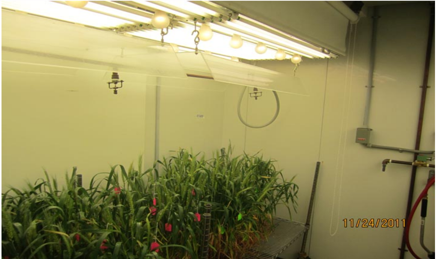
Cabinet misting system
